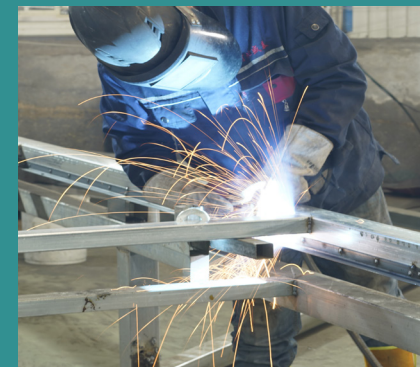
Floor frame welding
