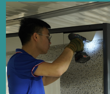
Wall panel assemble
